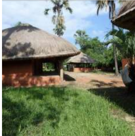
STAFF QUARTERS (SINGLE ROOMS) AROUND A CENTRAL REFECTORY WITH SHOWERS AND LATRINES.
