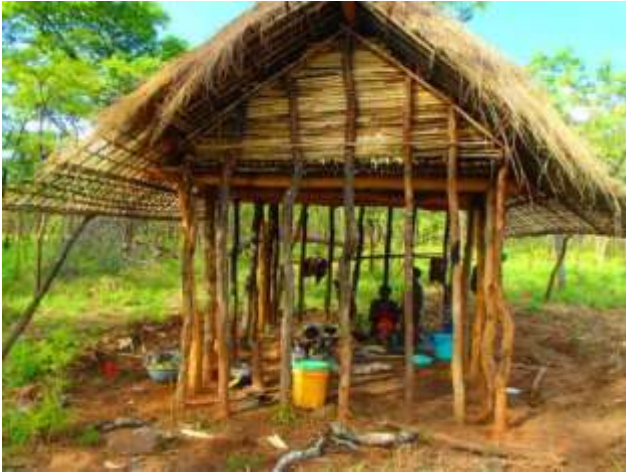
SAFE SHELTER FROM THE GUARDIAN FROM GOMBA VILLAGE – NOTE SLEEPING AREA ON STILTS
